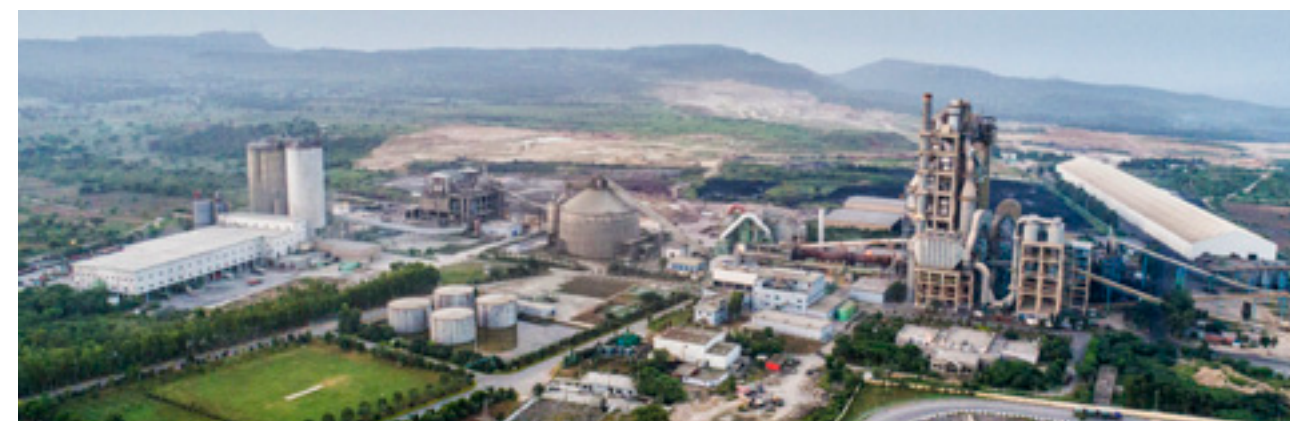
Bestway Cement, Kalar Kahar plant
